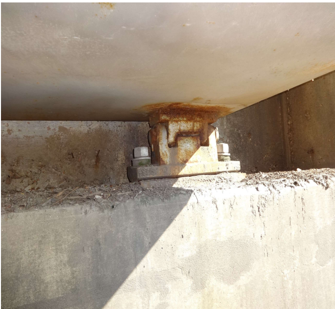
PHOTO 1 Description Rust on bearing assemblies & to outside bottom of all girders at Bearing assemblies at Abutment 1 & 2.
