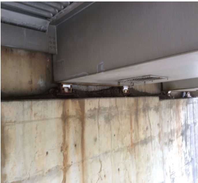
PHOTO 1 Description Debris on cap @ Abutment 1.
