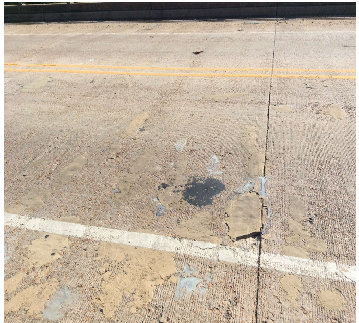
PHOTO 2 Description Spalls with no rebar exposed to deck at Spans 1 & 2.
