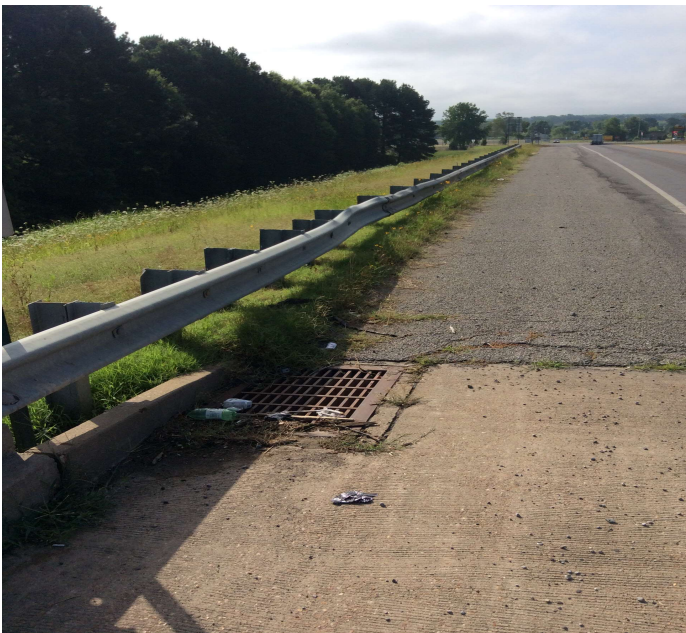
PHOTO 1 Description 10' of left approach rail is bent at Abutment 2.
