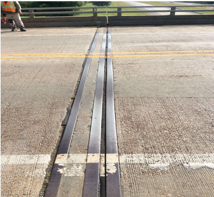
PHOTO 1 Description Adhesion failure to joint seal at Abutment 1.
