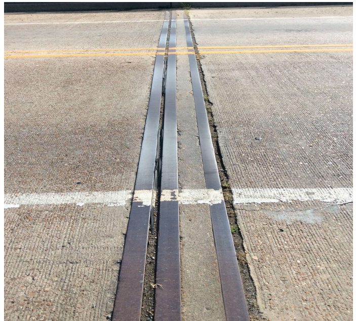
PHOTO 2 Description Joint seal is cracked & deteriorated at Abutment 2.
