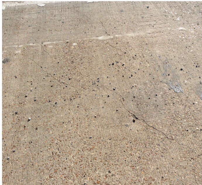
PHOTO 1 Description Unsealed cracks in deck at Spans 1 & 2.
